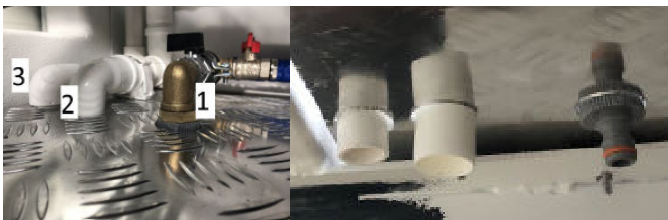
Figure 12 - Water and sewage connections with heating cord
