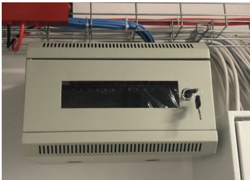
Figure 10 - Patch-panel box
