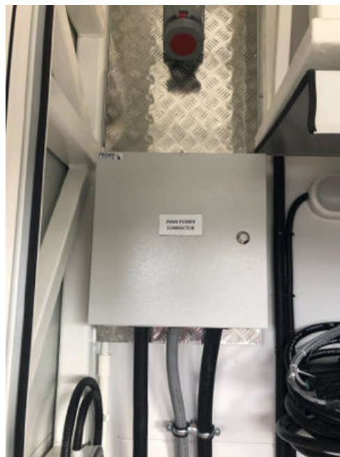
Figure 6 - Main power connector
